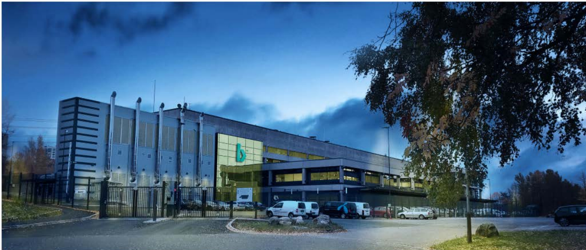
Bulk's data center in Oslo: Oslo Internet Exchange (OS-IX) in Oslo. Easy access to International Highways, railroad and International airport.
