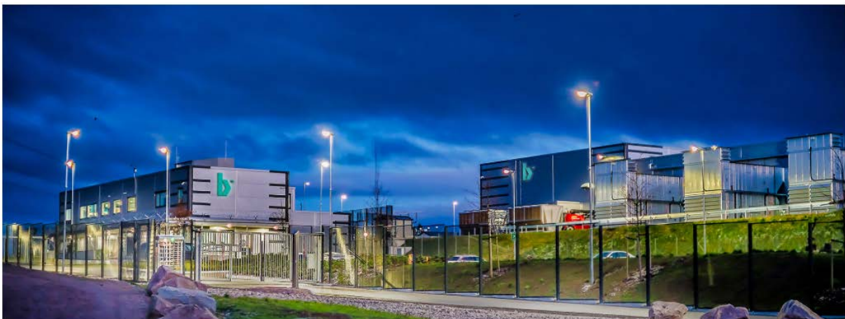
Southern Norwegian termination point: Carrier neutral Data Centers at Bulk's ultra-scalable N01 Campus outside city of Kristiansand, Norway.
